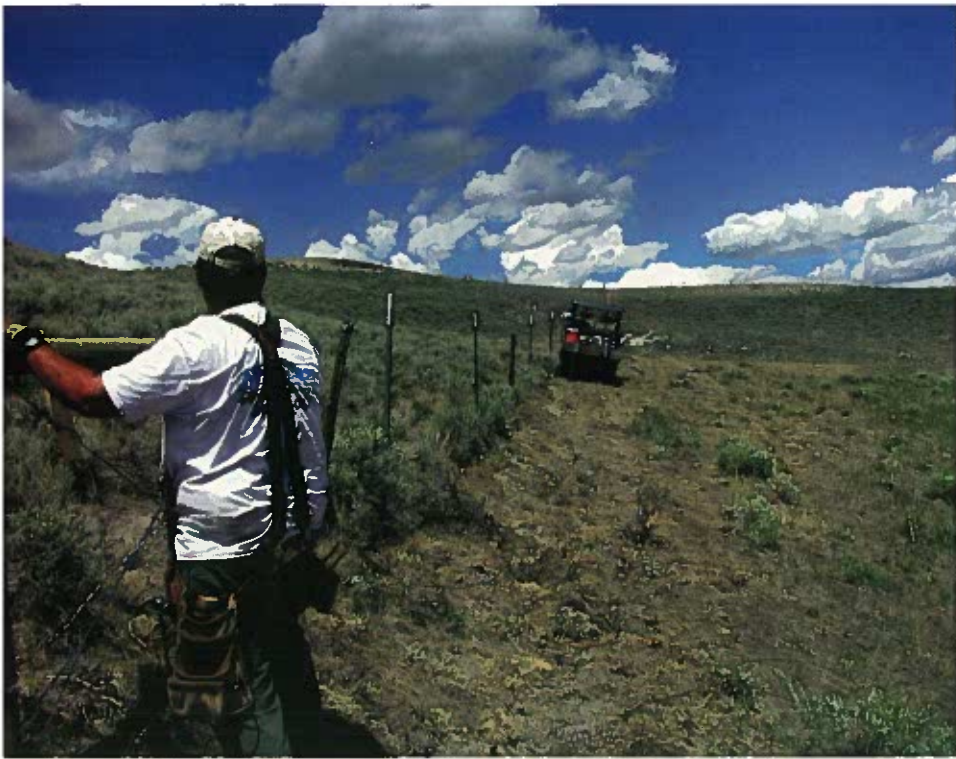
Installing improved fencing for migrating animals.
